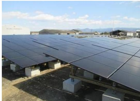
CIS thin-film solar modules installed on frame built with Japanese lumber
