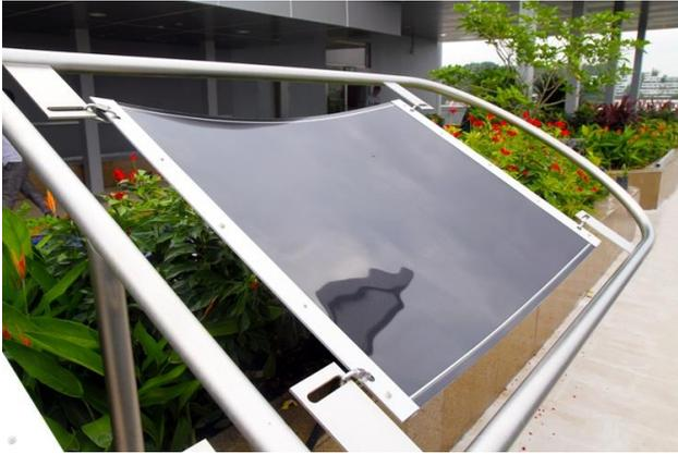
Photo: Solar Frontier's Prototype Ultralight and Bendable CIS Modules installed at PSA's new Terminal Building
