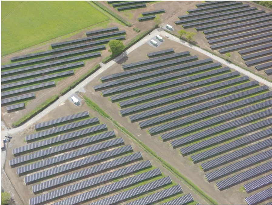
Photo: 7.15 MW Banwell Project, UK
